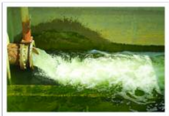
Recycled water effluent from San Jose Creek Plant.
