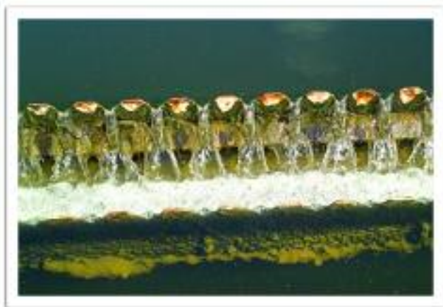
Settling Basin at San Jose Creek Water Reclamation Plant.
