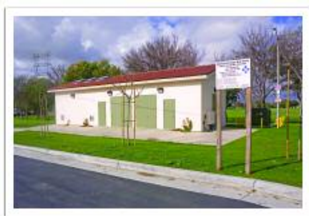
Hollydale Pump Station at Hollydale Park in the city of South Gate.
