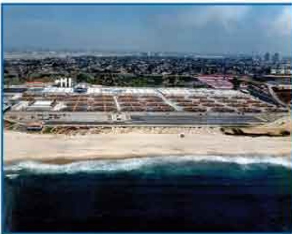
City of Los Angeles' Hyperion Wastewater Treatment Plant
