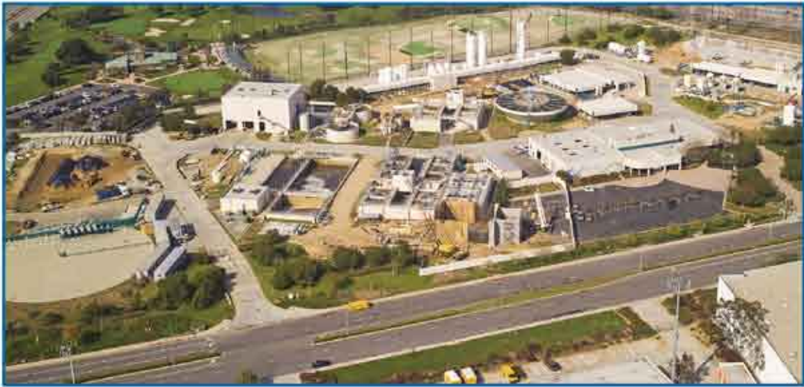
Figure 8-1 West Basin's Water Recycling Treatment Facility
