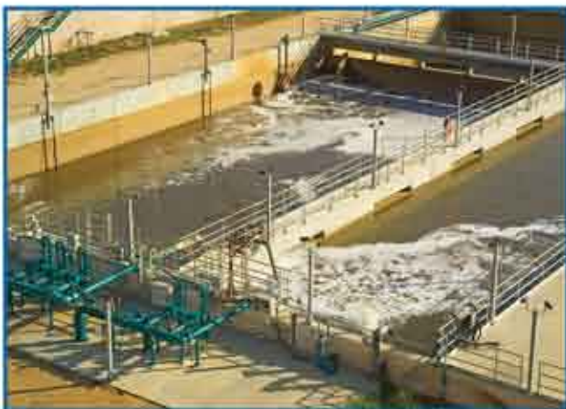
West Basin's Water Recycling Facility
